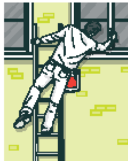
INCORRECT ✗ Overreaching and not maintaining three points of contact
